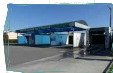
STATION DE LAVAGE LORIENT
